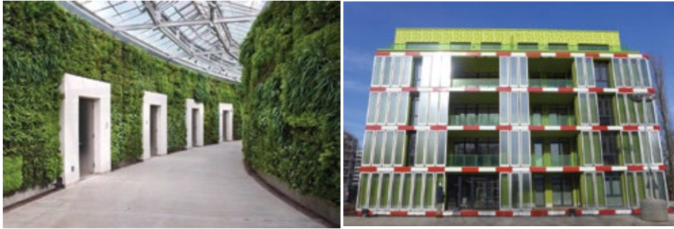
New “living” buildings that grow their own energy. Image Source Left: Victoria Lockhart PowerPoint, Global Wellness Summit 2016 Right: The BIQ house in Hamburg, Germany, the world’s first project to showcase a bioreactive façade (using embedded microalgae) to grow its own energy (Source: ARUP)
